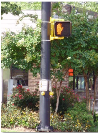
Existing pushbutton signal at the Square
